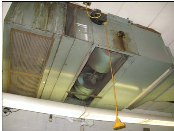
Indoor Air Handling Unit Horizontal Configuration Suspended by Structure Above
