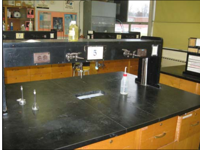
Science Lab Work Tables with Natural Gas Turrets
