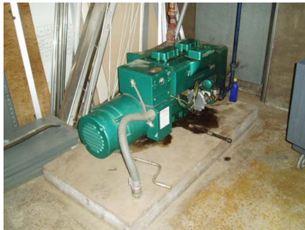
Figure E-4. Upper Level Generator
