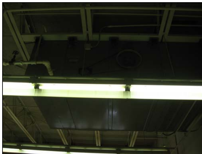
Indoor Air Handling Unit Horizontal Configuration Suspended by Structure Above
