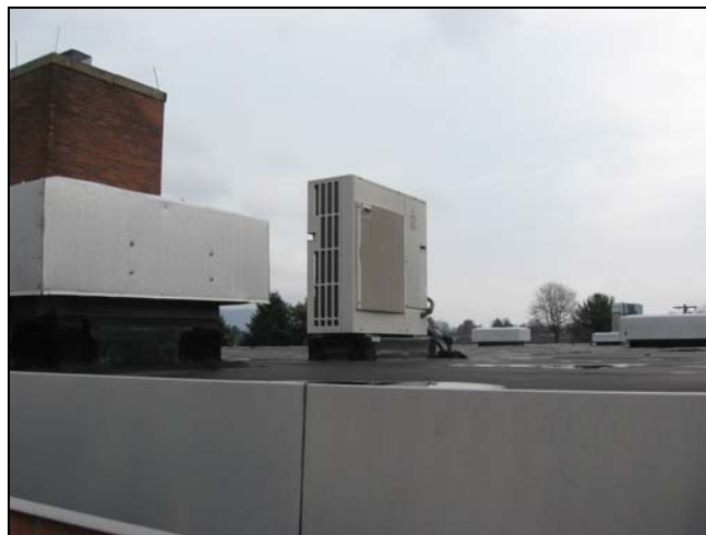
Outdoor Section of Ductless Split System
