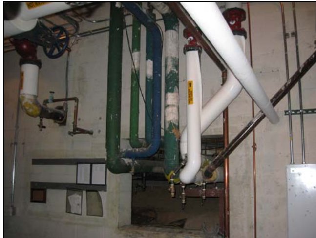
Piping Entrance into Crawlspace
