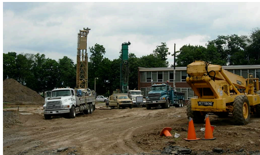
Geothermal well drilling begins at FTES
