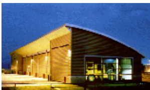
Snow Removal Equipment Storage University Park Airport
